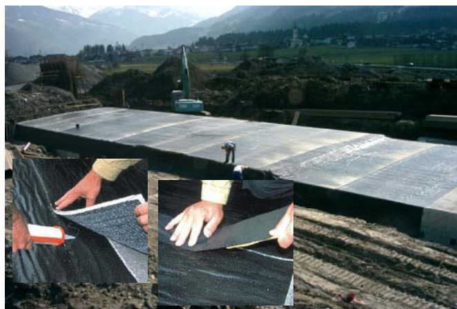
Offene Bauweise, Tunnelabdichtung Cut and cover technique, tunnel sealing
